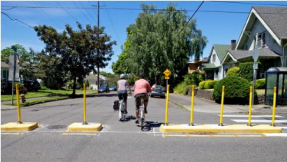
Flex post quick build diverter in Portland
